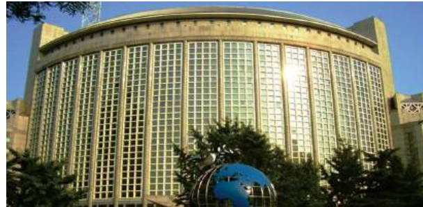
State Security Bureau Jinge Lou Data Center
