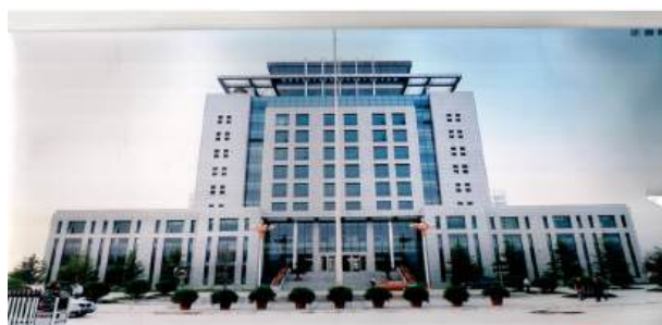
Guangdong Taxation Bureau Data Center
